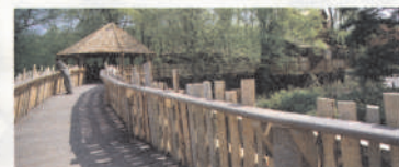
Top left: The DDA-compliant timber ramp bridges the levels between the ground and the treehouse.
